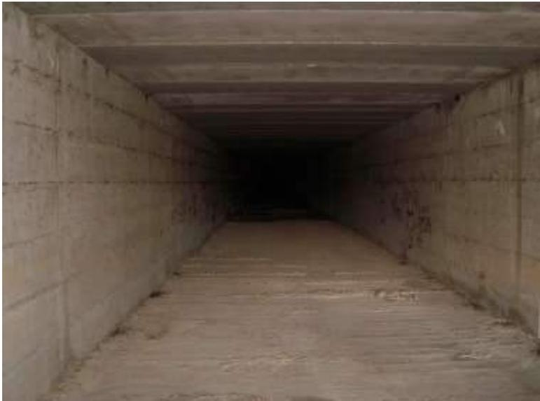
A photograph showing the interior of a long, narrow buried channel. The walls and ceiling are made of concrete. The floor is also concrete and appears to be slightly elevated from the surrounding ground level. The channel is empty and leads into a dark tunnel.                                              |
